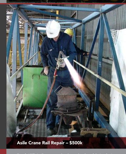
Dual 40T Asile cranes had cracked welds in their support structure. Detech Engineering determined the most appropriate solution (thermit welding) and developed / designed / trialled an access system mounted to the cranes to complete the works.
